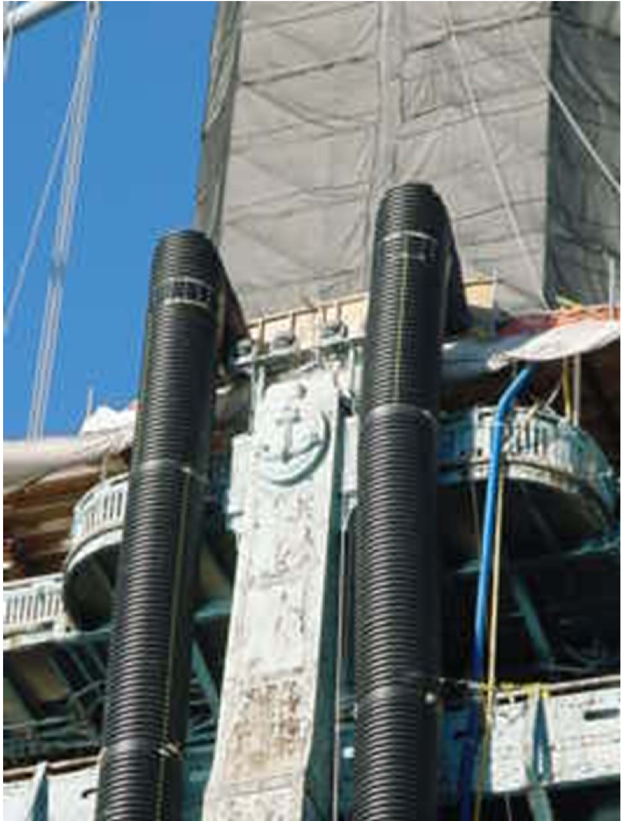
Ben Franklin Bridge Tower – Exhaust Ducts
