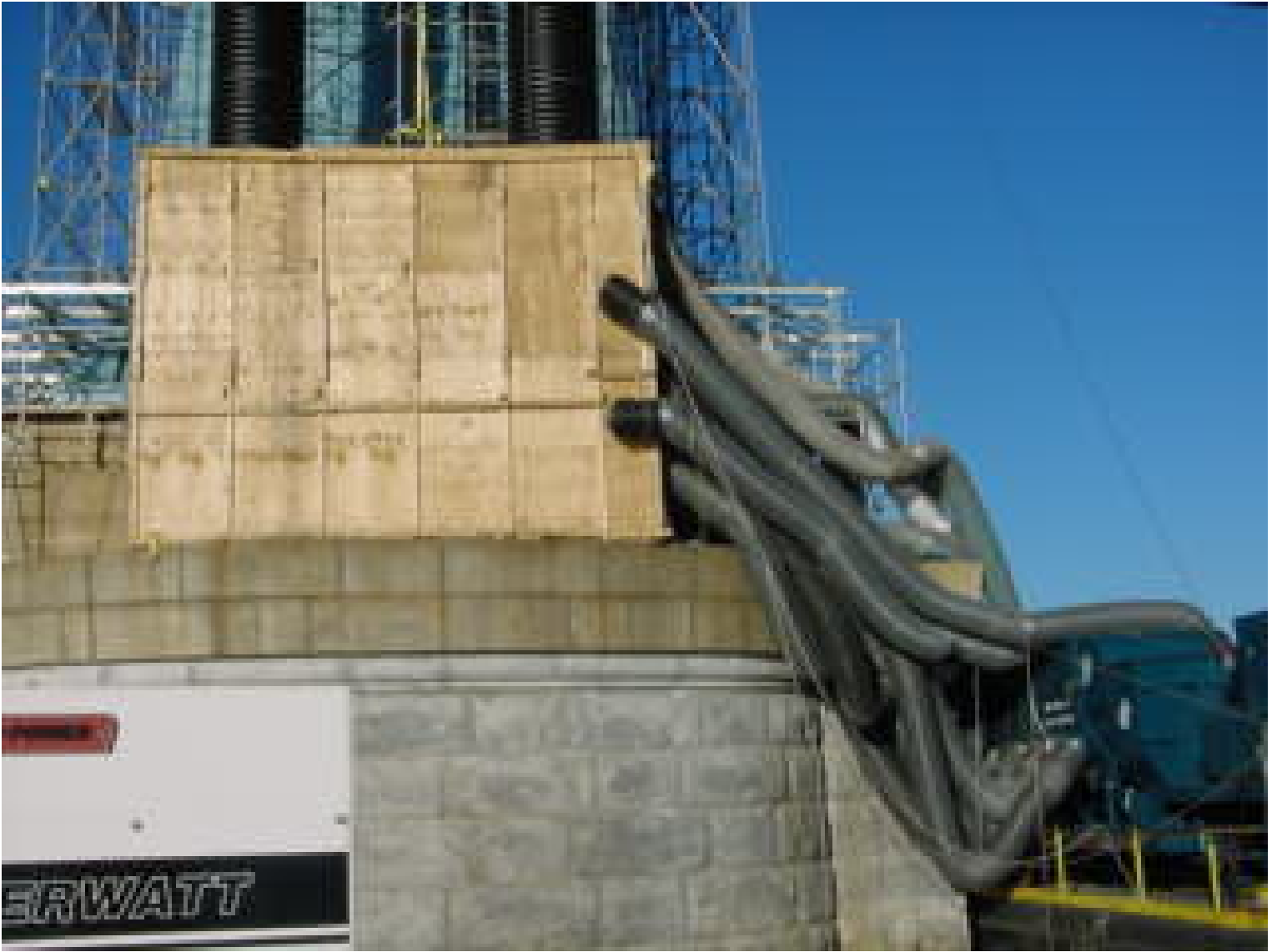
Ben Franklin Bridge Tower – Exhaust Ducts From Dust Collector
