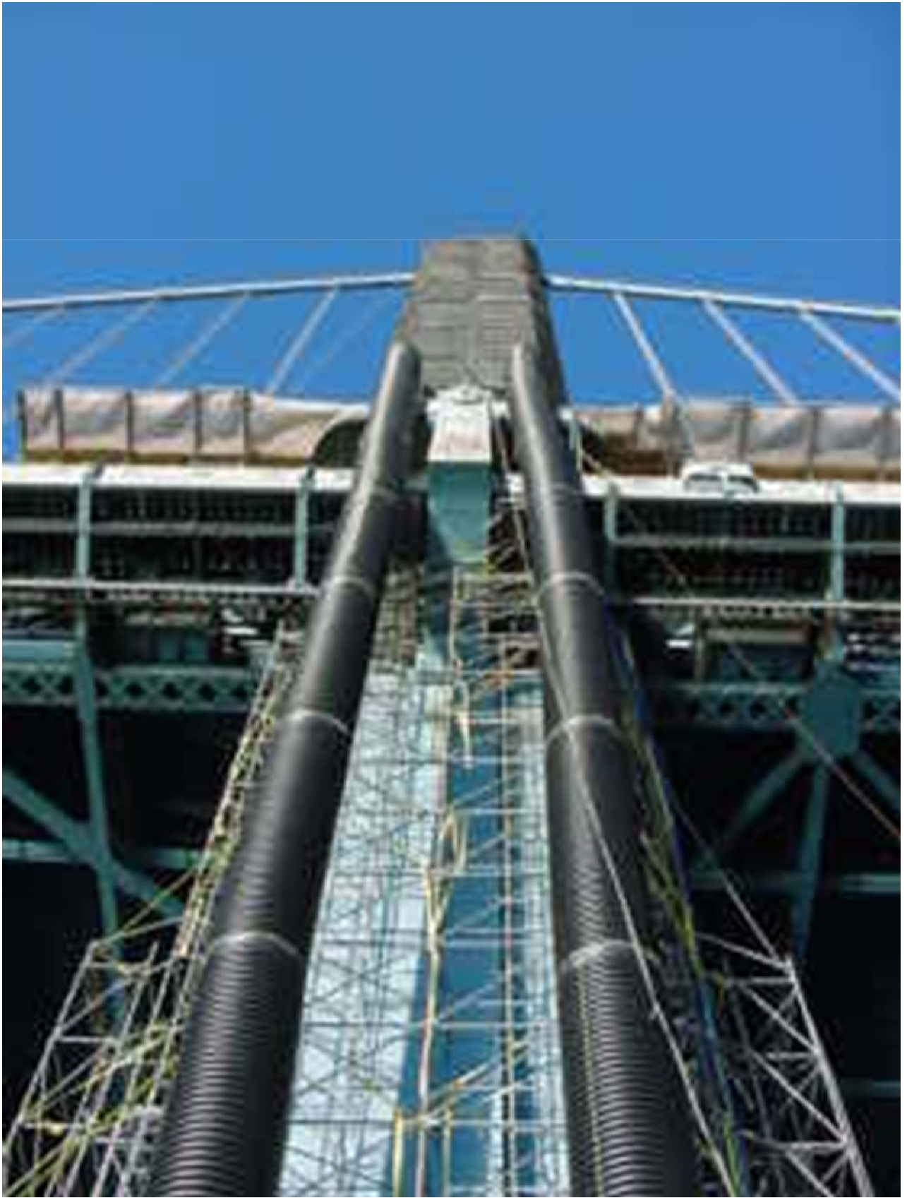
Ben Franklin Bridge Tower – Scaffold Supported Exhaust Ducts
